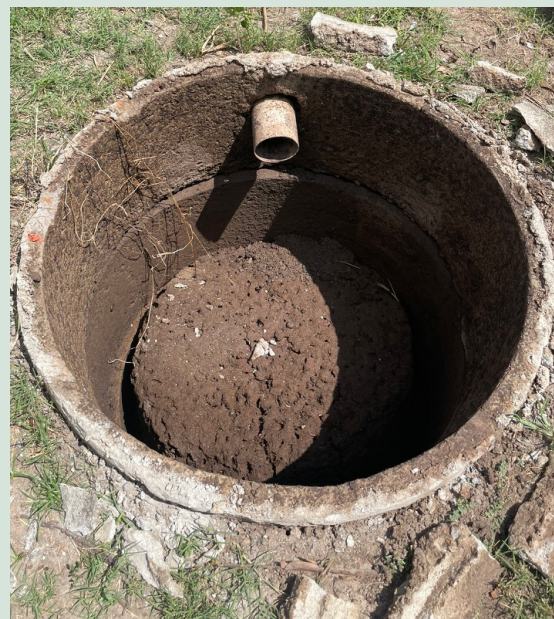
Local team and beneficiary showcasing the successful opening of a toilet's owner pit including decomposed faecal sludge (below)
