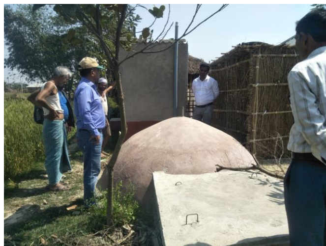
Figure 6: Toilet Linked with Bio-digester
