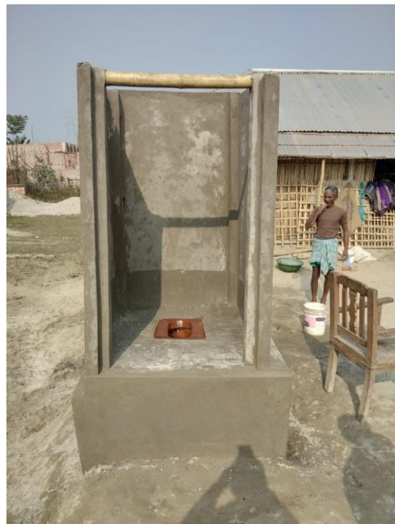
Figure 8: Pakka Super structure made the beneficiary
