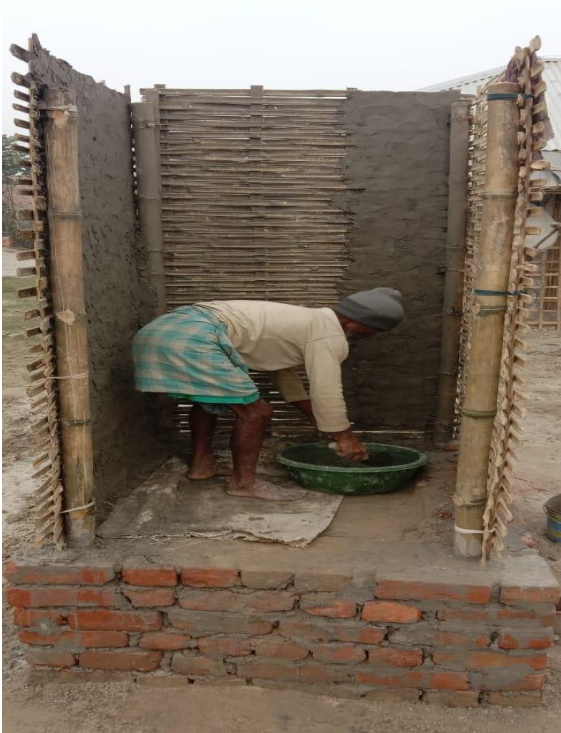
Figure 8: Low-cost bamboo super structure
